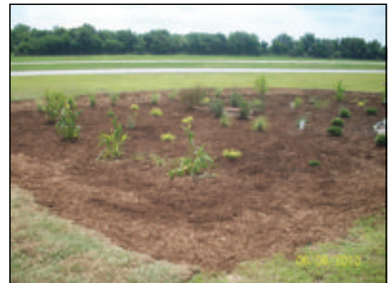
Newly installed rain garden at Owens Field Airport.
