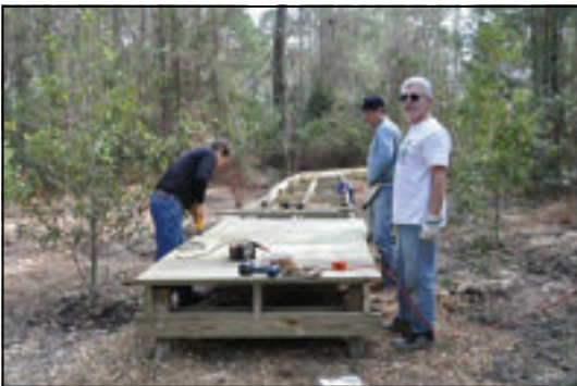
Volunteers build a boardwalk for the Tree of Life rain garden.
